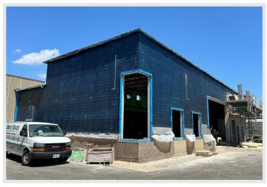
Findorff masonry crews working around the Skills Lab Addition installing brick veneer and cast stone units. Looking sharp!
